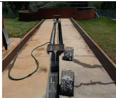
Figure 7-2: WWTW Inlet headworks
