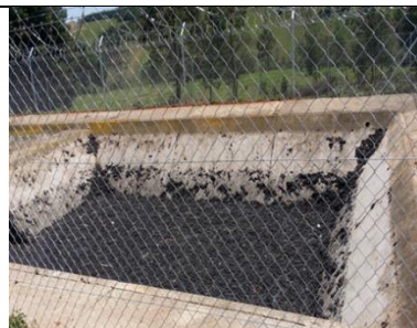
Figure 7-5: WWTW aerobic tank used as a drying bed
