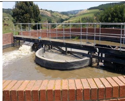
Figure 7-3: WWTW Settling tank
