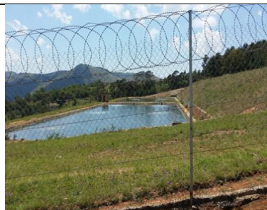
Figure 7-4: WWTW maturation ponds
