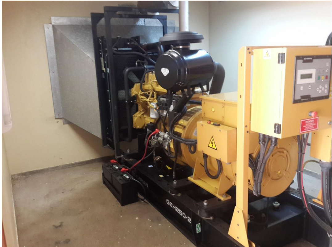
Figure 8-1: Diesel generator
